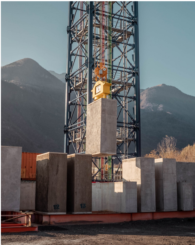
Above: As the jib lowers the blocks, the suspending cable drives dynamos to generate electricity. The blocks drop at about 3m/second and each generates around 1MW as it falls
